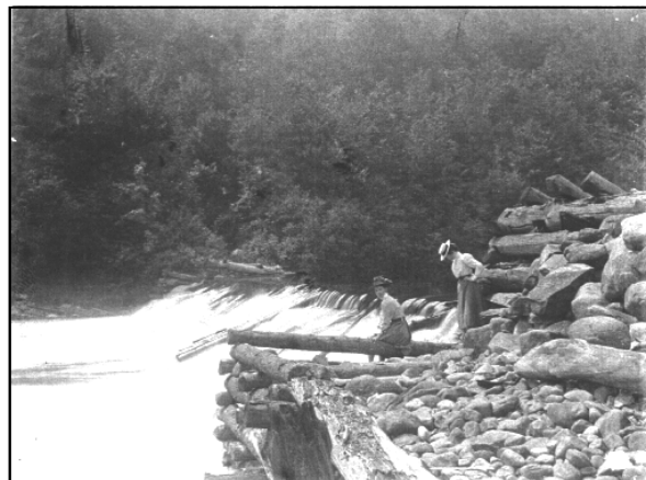
Hunters Creek Dam
